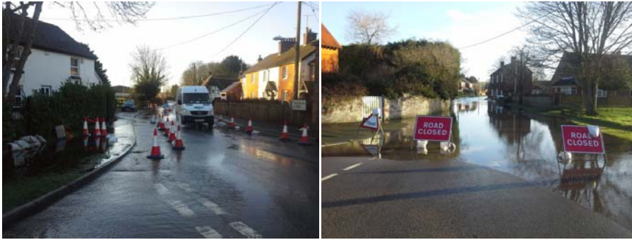
A number of roads in Wiltshire had to be closed or traffic movements restricted because of flooding in 2014.
